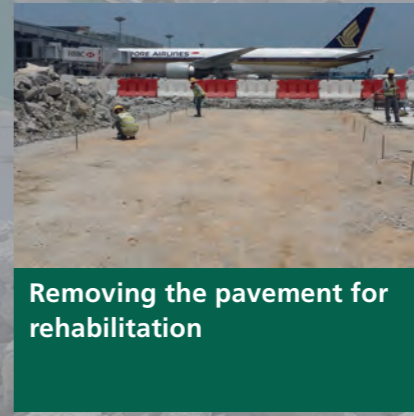
Aircraft parking bay restored with minimal new materials used
