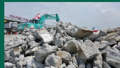
Demolition of existing rigid pavement
