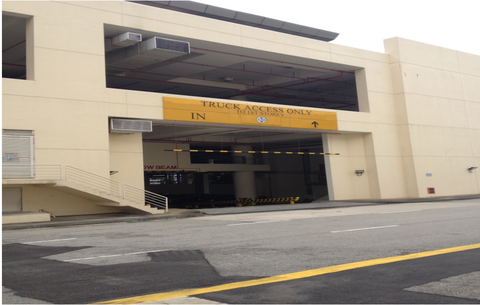
Truck entry point at Megaplex 1
